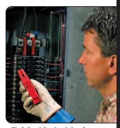
Find the right circuit breaker, sort and trace wiring
